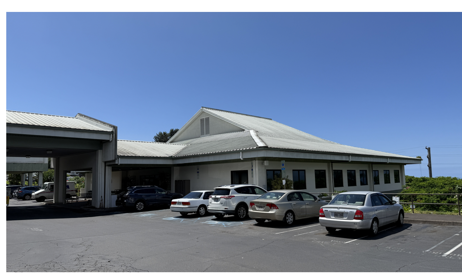
11 PHOTO REF - AREA D EAST AND NORTH ELEVATION A90 NTS
