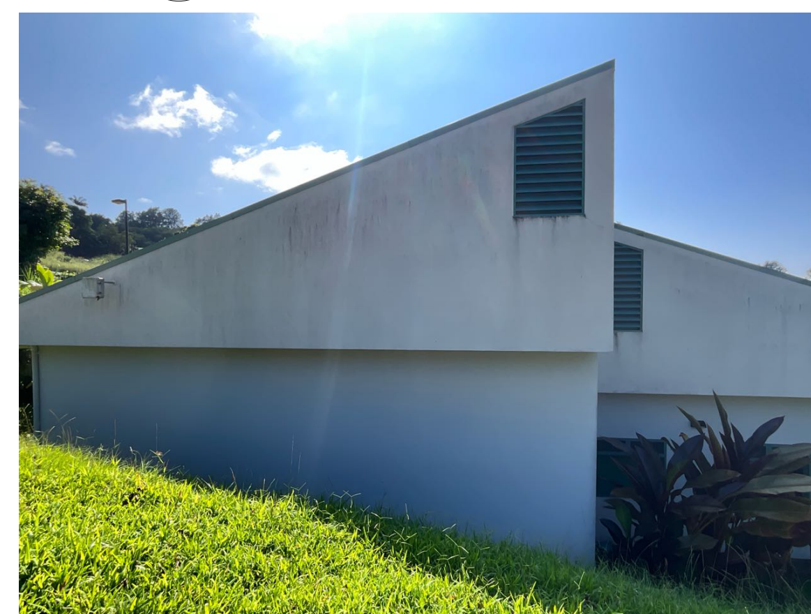
15 PHOTO REF - AREA E WEST ELEVATION A90 NTS
