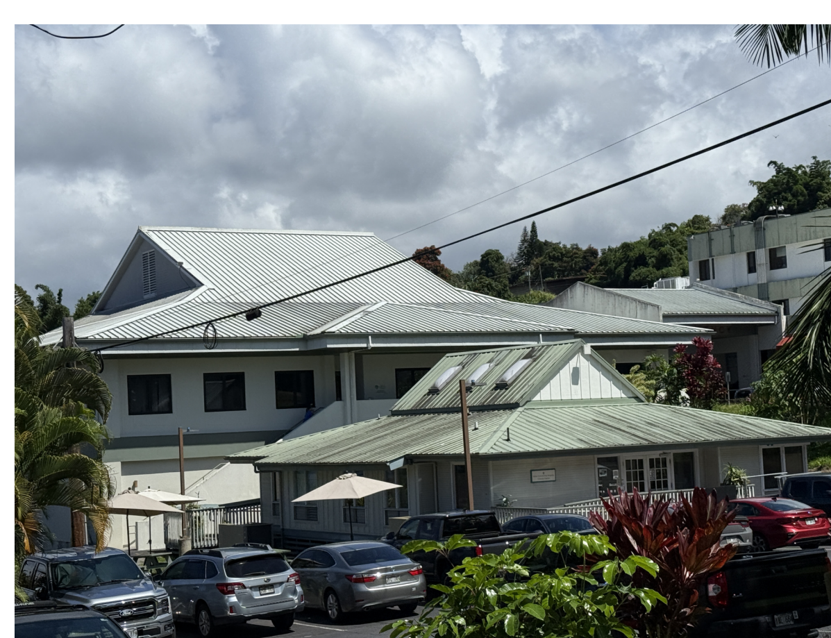
10 PHOTO REF - AREA D EAST ELEVATION A90 NTS
