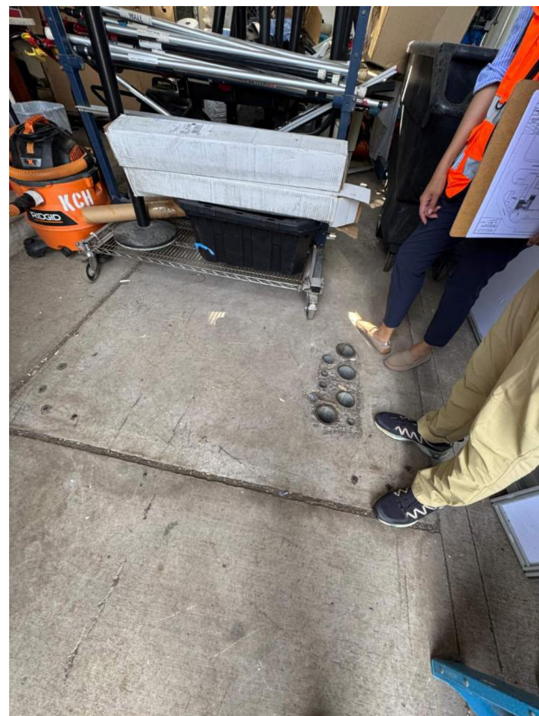
3 WAITING AREA - PENETRATIONS TO INFILL A92 NTS
