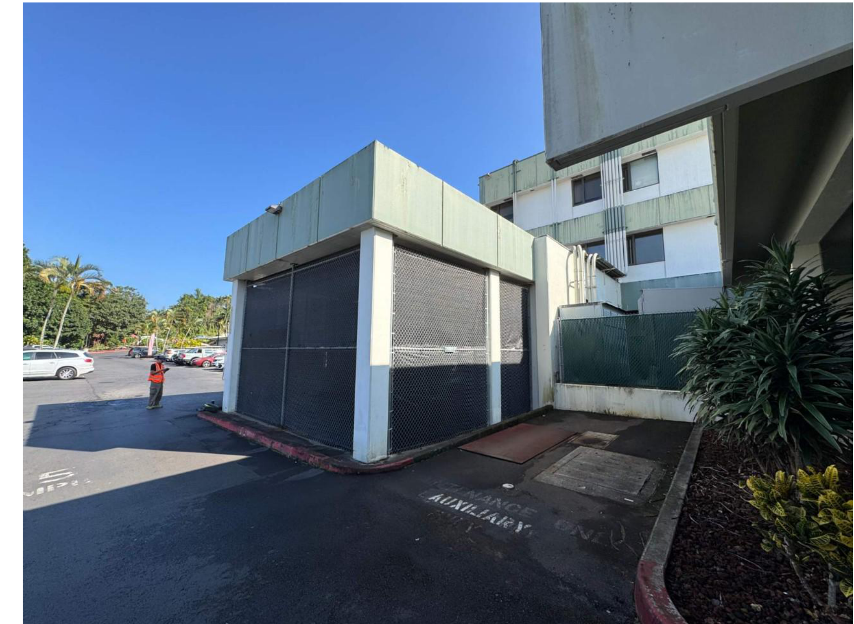
4 WAITING AREA - OVERALL PHOTO A92 NTS
