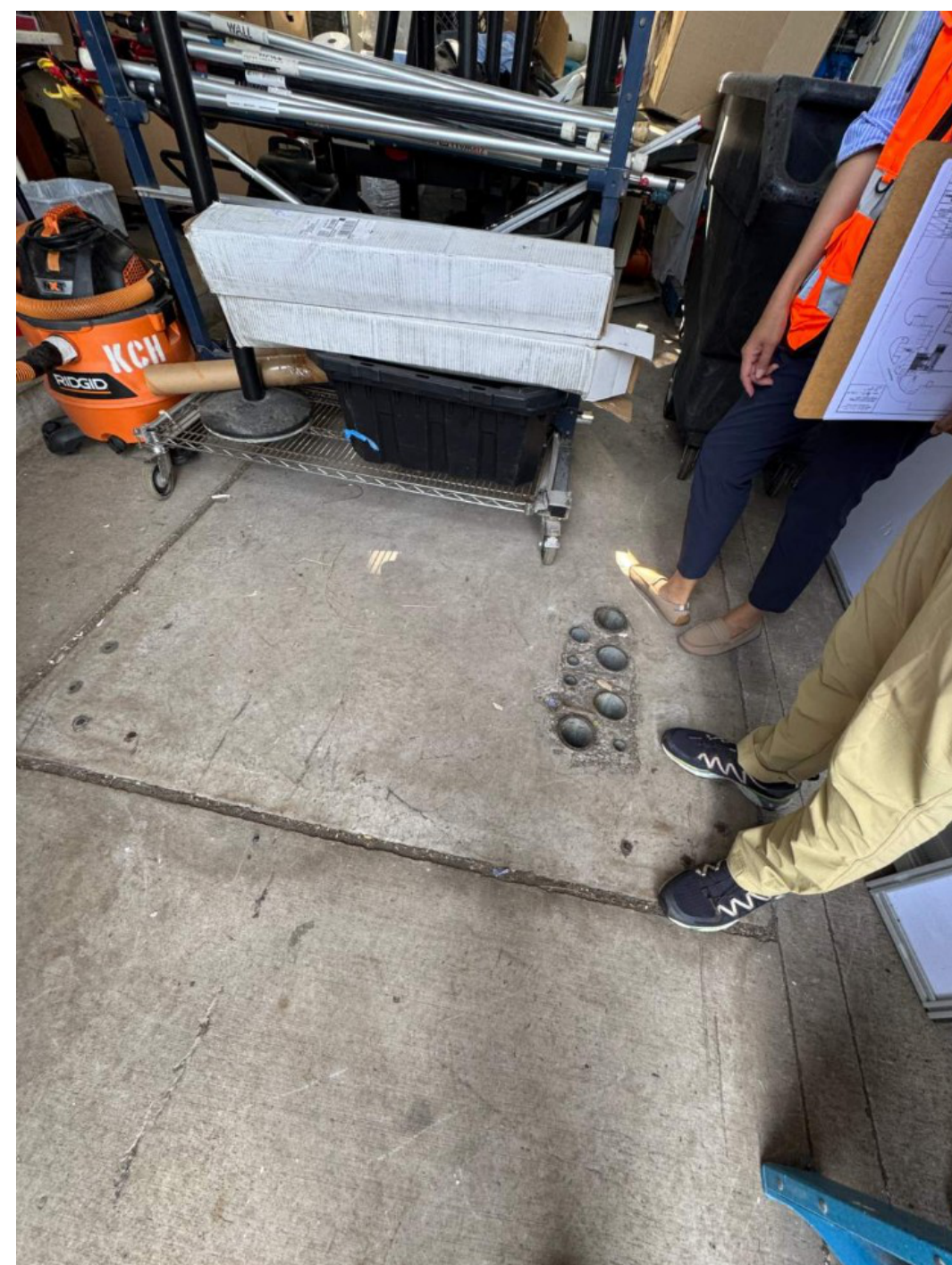
3 WAITING AREA - PENETRATIONS TO INFILL A92 NTS
