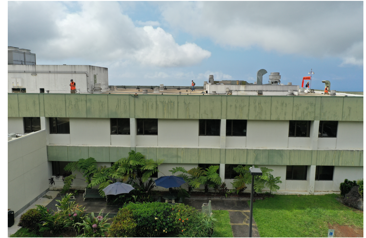
5 PHOTO REF - AREA B NORTH ELEVATION A90 NTS
