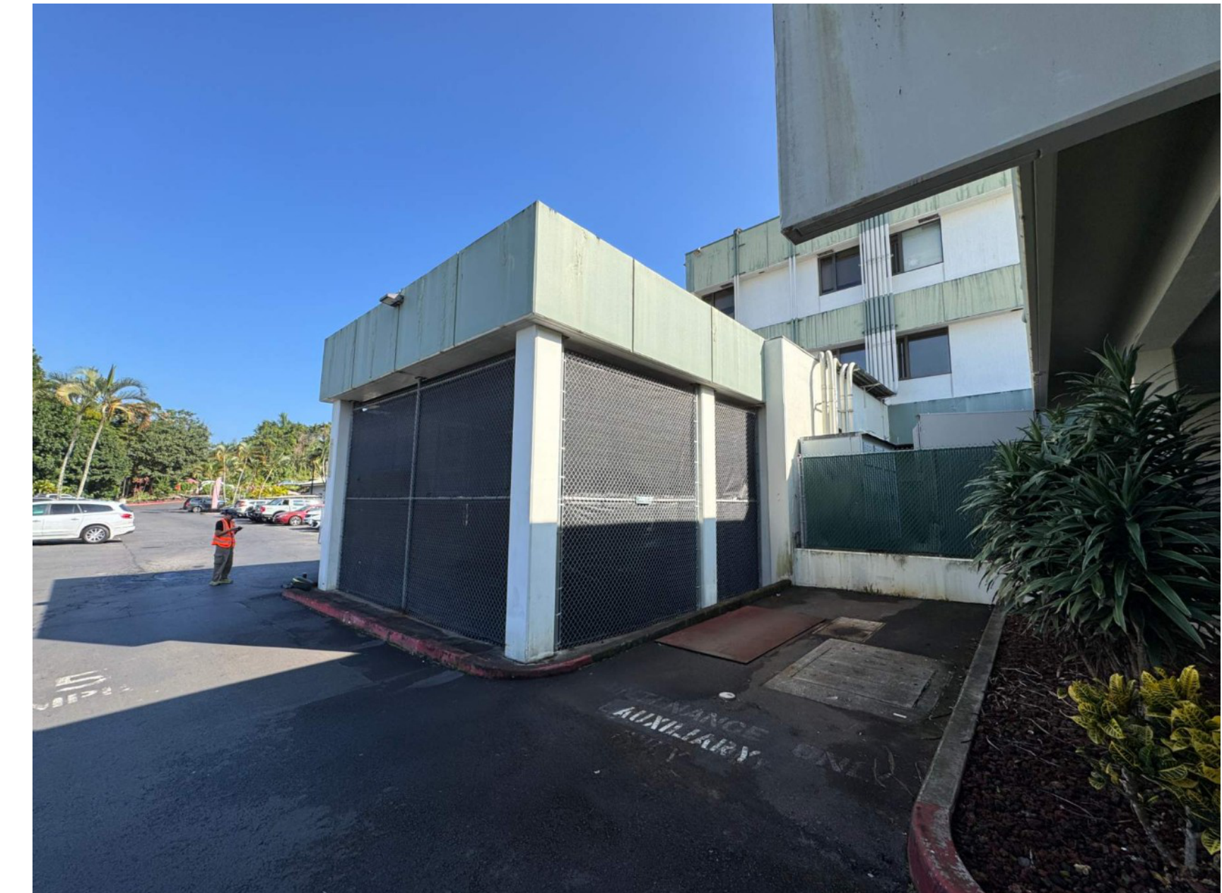
4 WAITING AREA - OVERALL PHOTO A92 NTS
