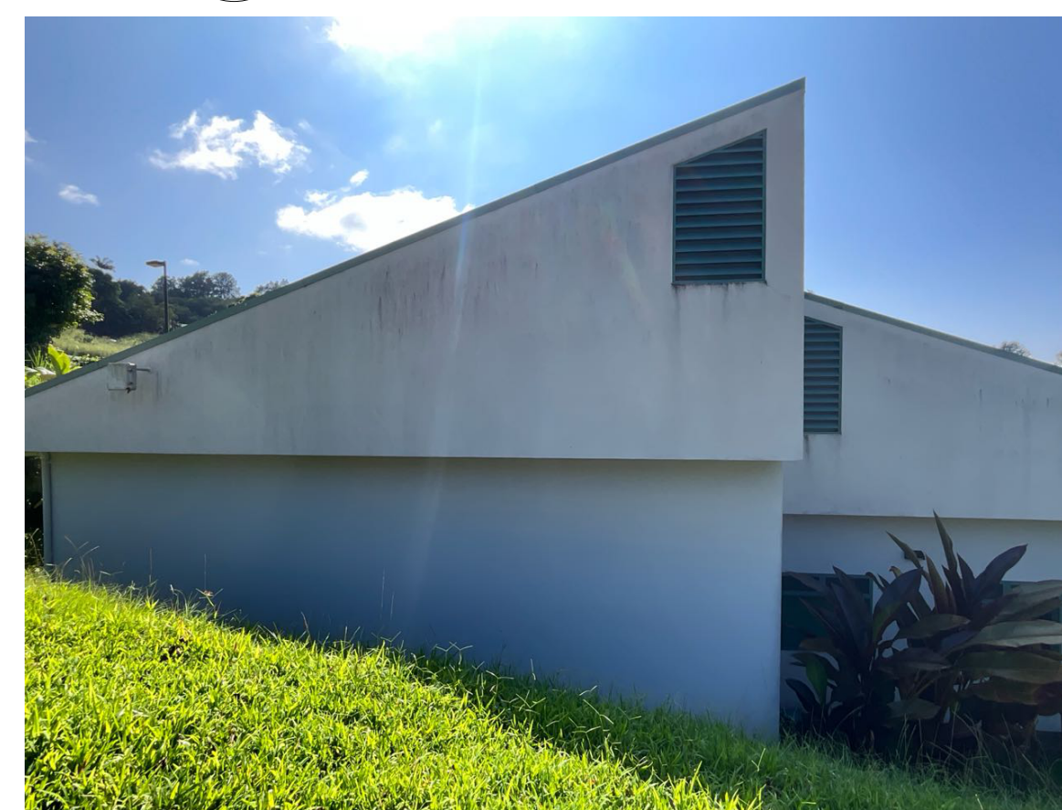
15 PHOTO REF - AREA E WEST ELEVATION A90 NTS
