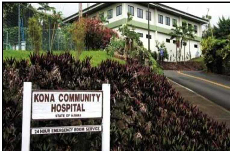
Kona Community Hospital Main Building November 2019
