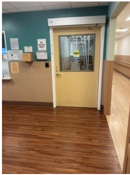
1. Looking from the Main ED doors to the FastTrack door
