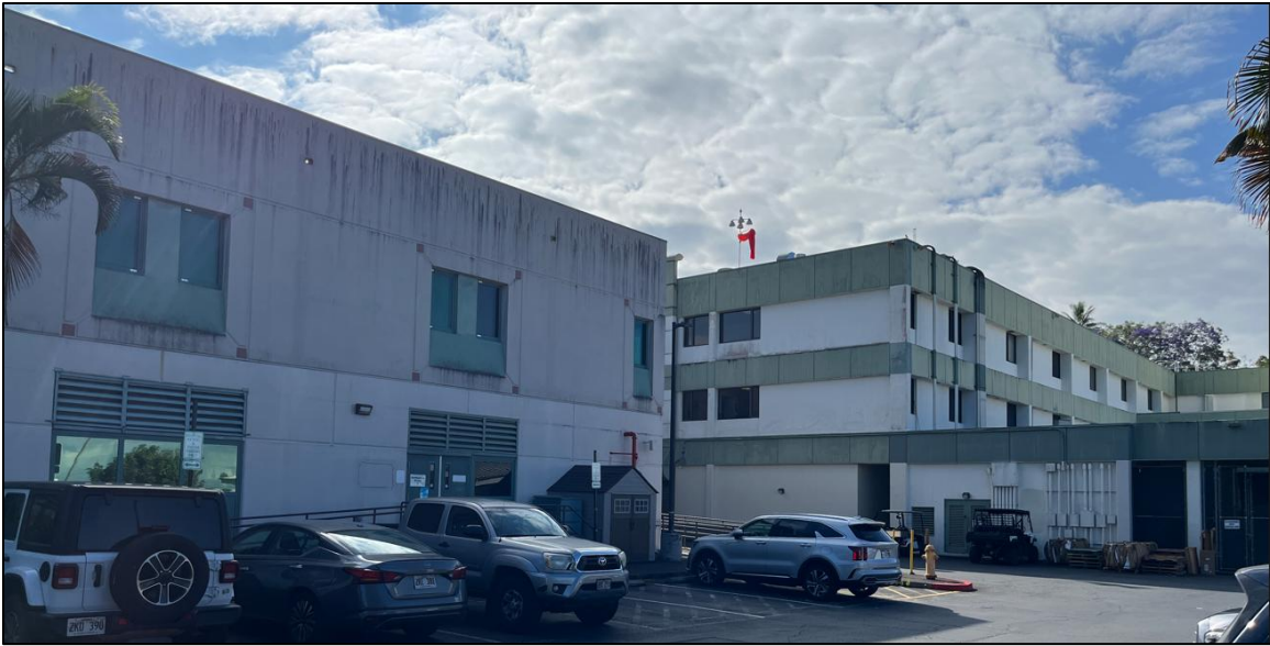
Photo 10 - Overview of Building 1 exterior walls and windows facing southeast
