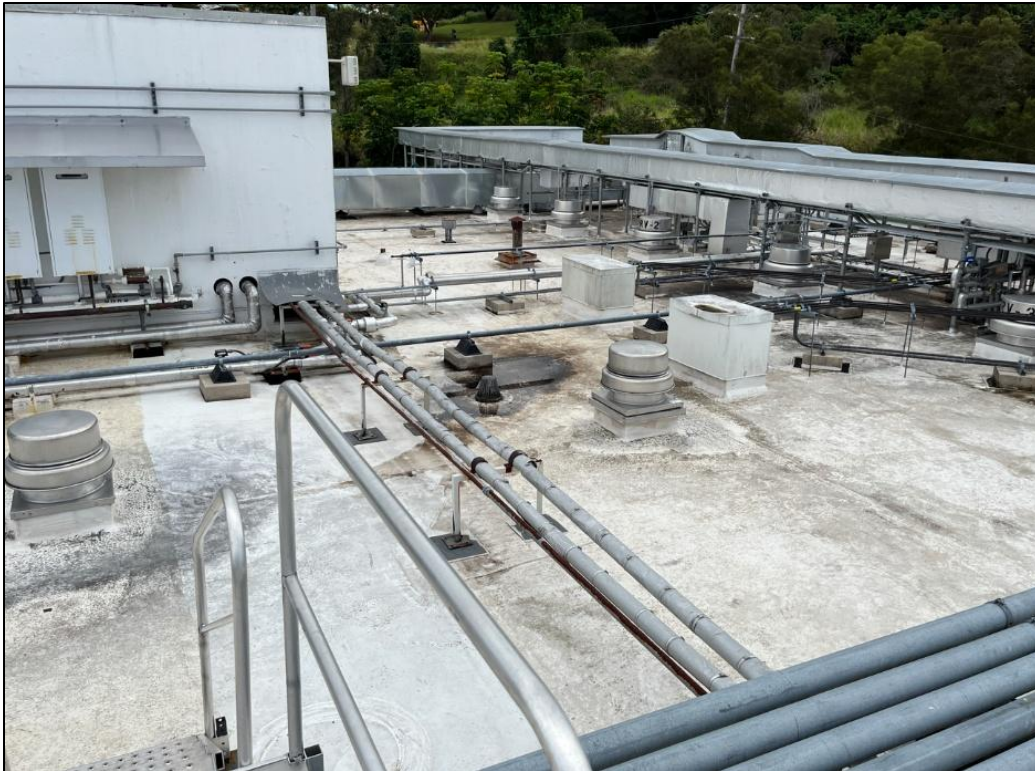
Photo 2 - Overall view of Building 1 low slope roof area facing southeast
