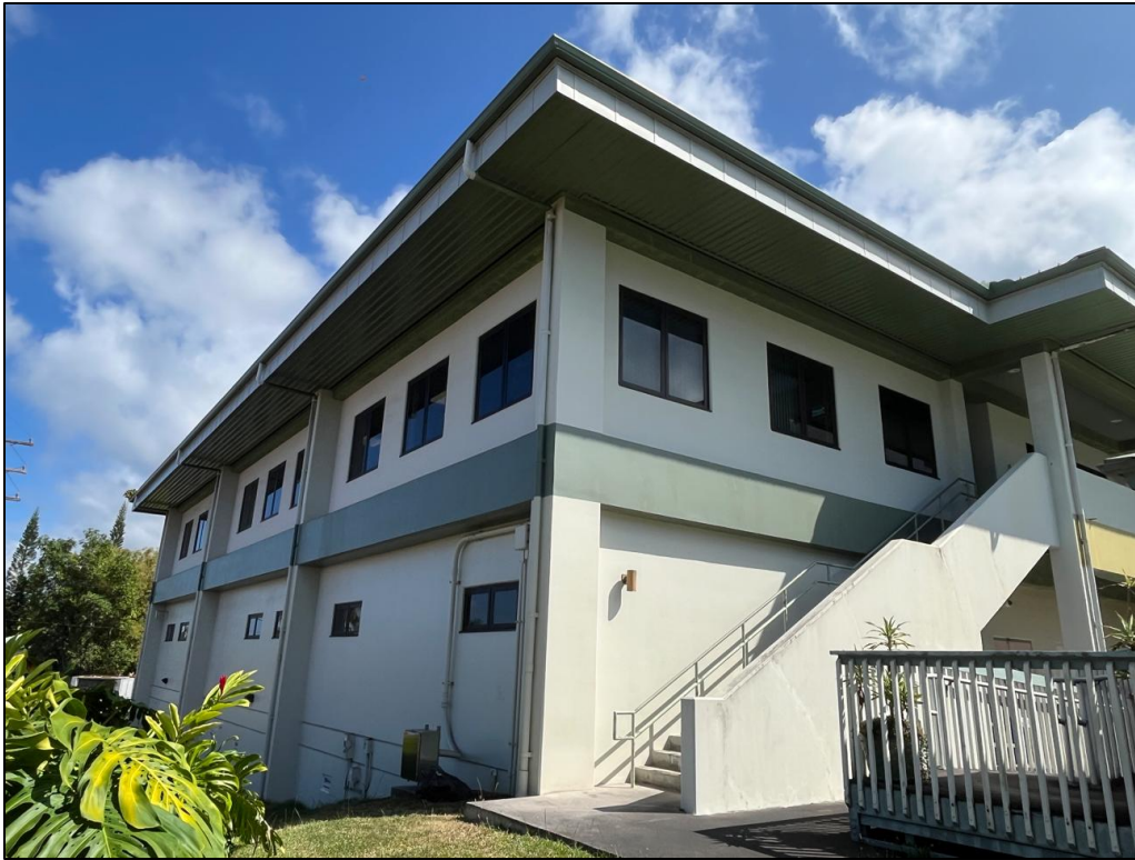
Photo 20 - Overview of Building 2 southwest elevation
