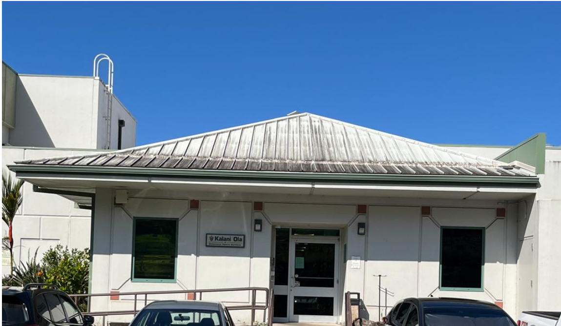
Photo 5 - Behavioral Health Services Building standing seam metal panel roof
