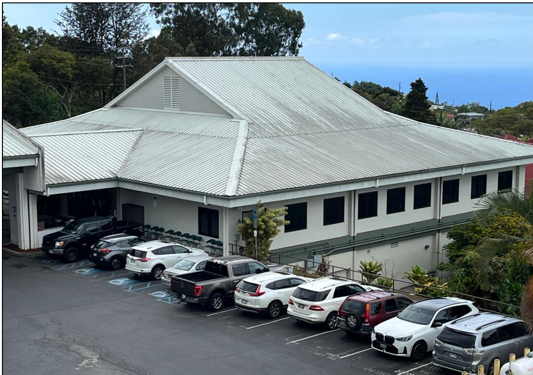
Photo 18 - Overview of standing seam metal roof at Building 2 (facing south)
