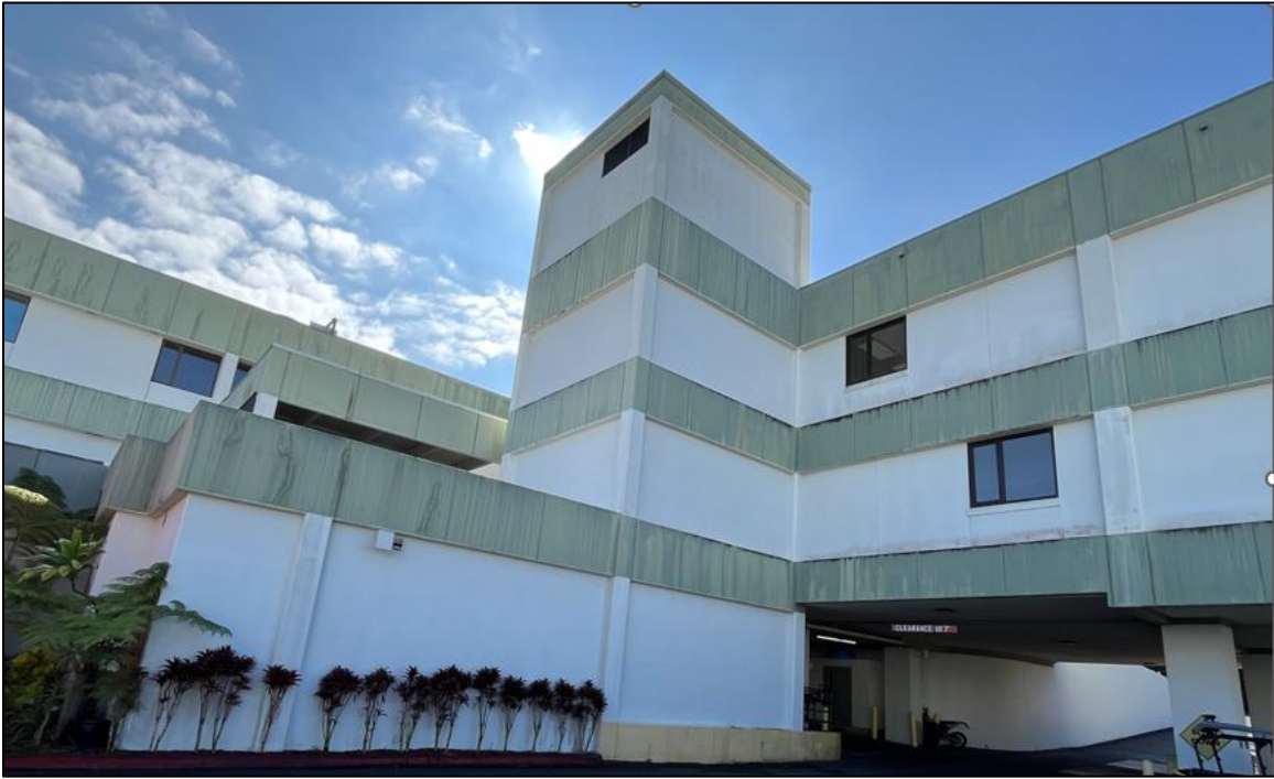
Photo 8 - Overview of Building 1 concrete walls typical condition
