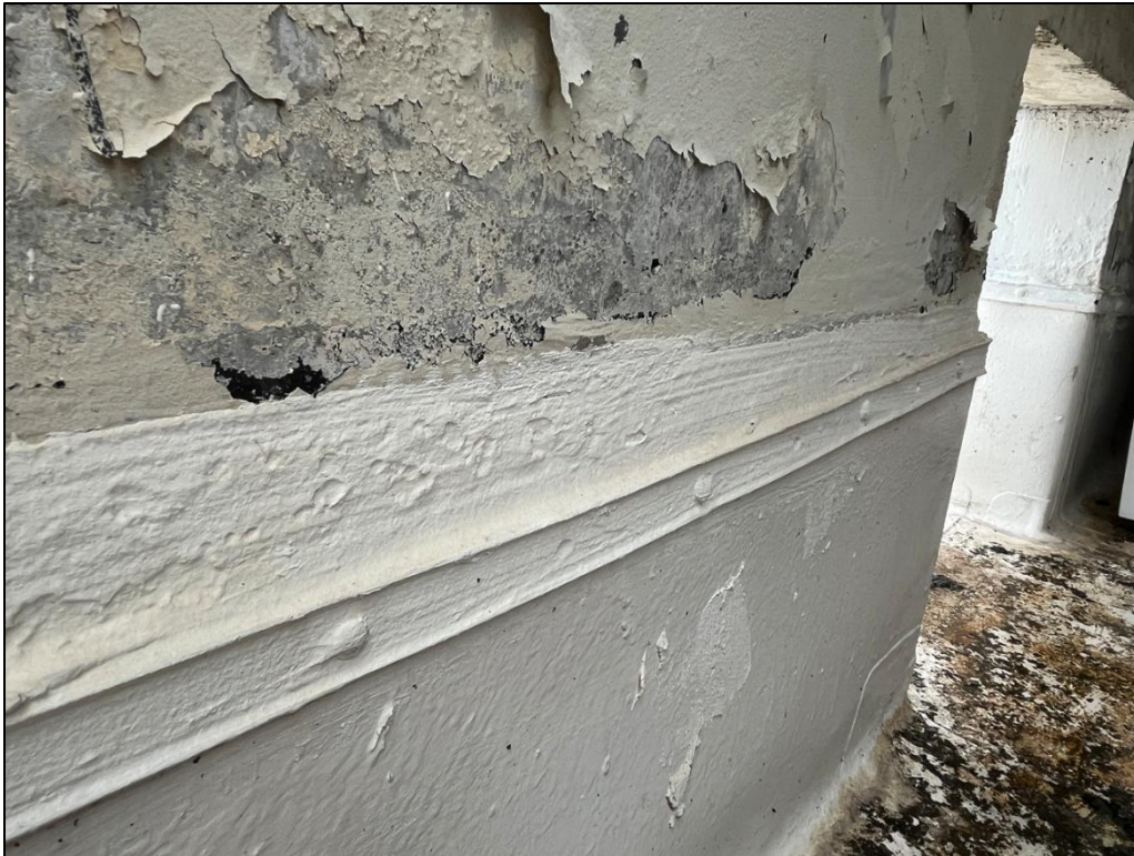
Photo 3 - Typical TPO membrane roof base flashing termination with fluid applied flashing repairs
