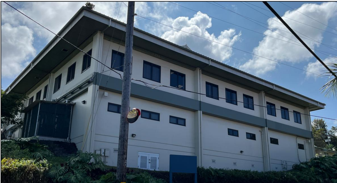
Photo 19 - Overview of Building 2 west elevation
