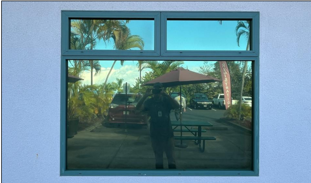
Photo 25 - Typical painted aluminum block frame window at Building 3
