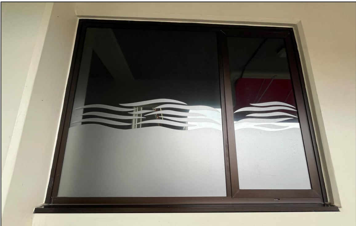
Photo 11 - Anodized aluminum block frame windows under porte-cochere at main entrance
